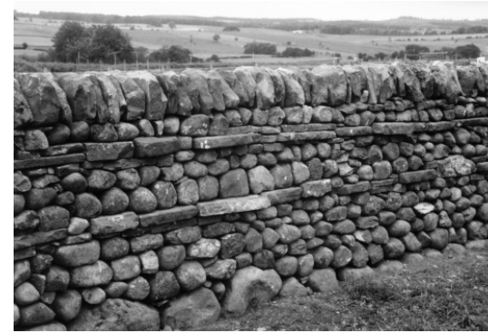
Complete bands of throughs, Langwathby, Eden Valley
