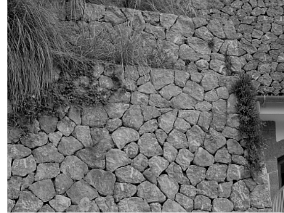
Retaining wall Sa Colabra, Mallorca © Sean Adcock
