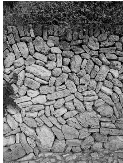
Retaining wall inside Capdepera fortress, Mallorca © Sean Adcock
