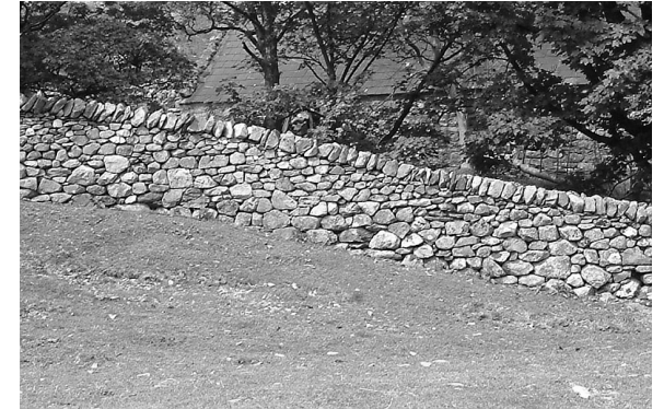
Above wall on slope showing jumpers and levelling. Left similar construction but on the flat. Both Blaen y Nant, Nant Ffrancon. Both © Sean Adcock
