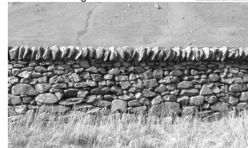
Above wall on slope showing jumpers and levelling. Left similar construction but on the flat. Both Blaen y Nant, Nant Ffrancon. Both © Sean Adcock
