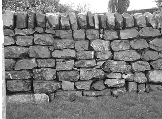
Joints and stacking, Anglesey. © Sean Adcock
