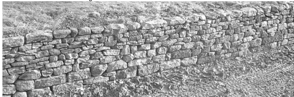
Random wall built from regular stone on a slight slope including pronounced short sections of regular coursing. Little Everden, Northamptonshire. © S.Adcock
