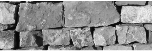
Fig.3. However you shuffle the oversized stones along there will be jointing issues
