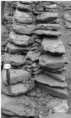
Slate waste and fines 'poured' into wall ©Sean Adcock
