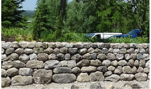
Fig.1. Here attempting to sit \frac{1}{2} on \frac{1}{2} has led to a ‘mushrooming’ of longer stones towards the centre of the section shown and a unbalanced structure compared to either
