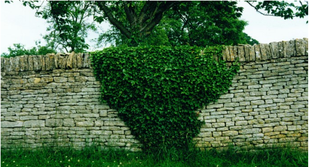
Fig.4. Random Coursed wall. Chilton, Oxfordshire
