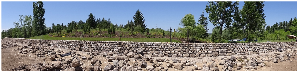
Fig.11. Varying the thickness of the top 2 courses is not necessarily obvious when viewed from more than a few metres away.
