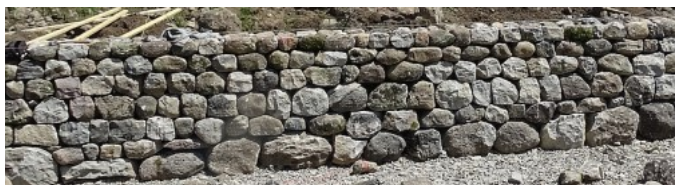
Fig.12. Random footings in a coursed wall
