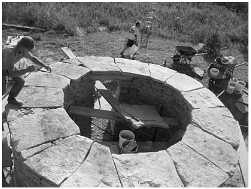
Eve plates on Cabane built at 4 th Canadian Rocktoberfest run by DSWAC ©John Shaw-Rimmington
