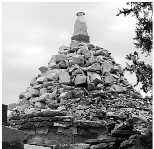
Finished trulli cone/dome awaiting tiling © Evan Oxland
