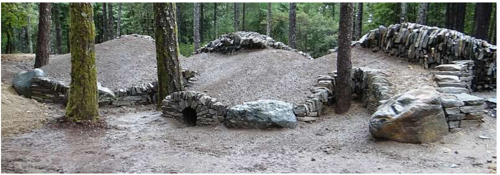
Fig.15. Back of the Wing wall (2)
