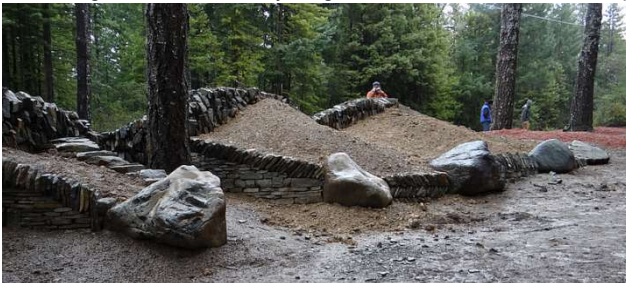
Fig.14. Back of the Wing wall (1)
