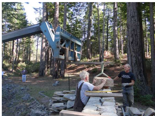
Fig.6. JSR and David setting a capstone with the help of the Gradall (and Peter of course)
