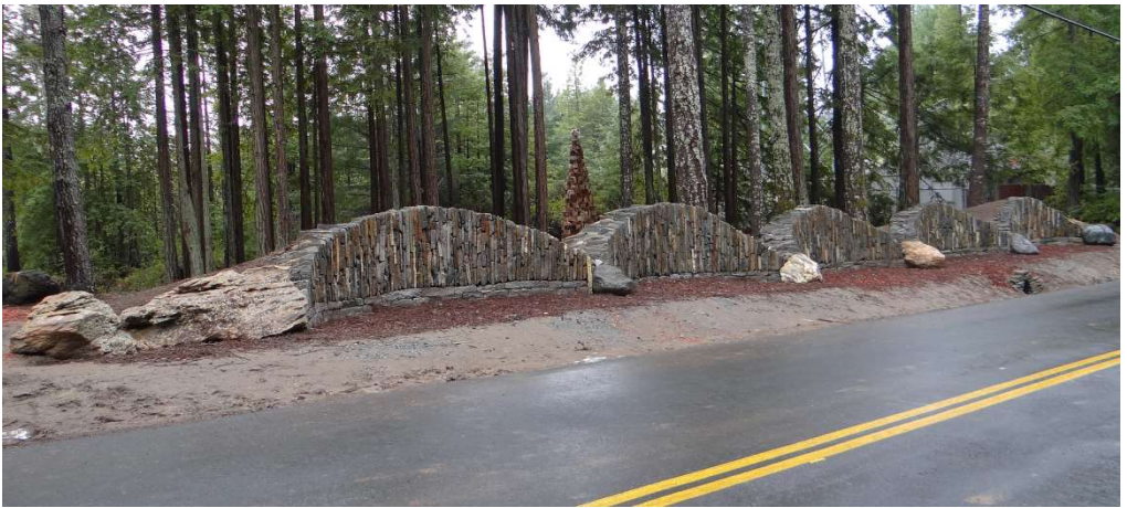
Fig 12. The completed wing wall
