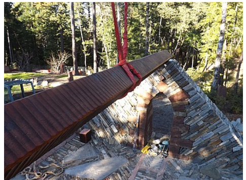
Below: The Beam is lifted into position Photo ©John Shaw-Rimington
