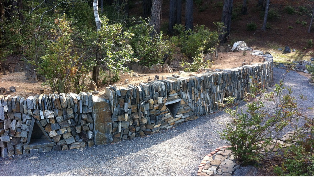
Wedge wall transforms from stacked wood to vertical slabs either side of yet another triangle.
