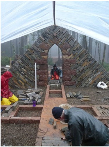
The 'paths' under construction. JSR Foreground Young Sean left, Dave at back Below JSR fitting yellow sandstone blocks
