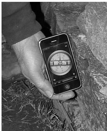
i phone with digital level being used to show an inverse batter.
