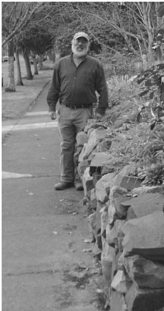
As can be seen here a severe bulge is a fault in both line and batter.
